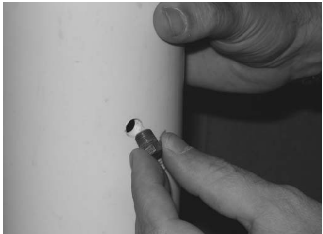
Figure 9.3: Insert Pipe Plug into Test Port
